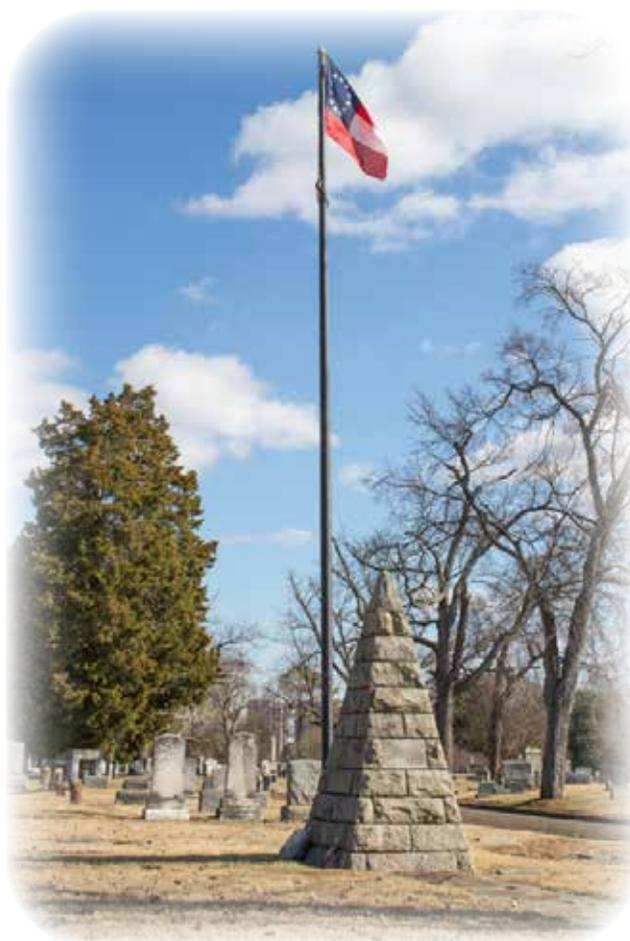
stones together has begun to crumble with age and fall out, leaving the internal structure exposed to the elements, particularly water when freezing and thawing can cause the stones to crack. Likewise the concrete work around the plot has
